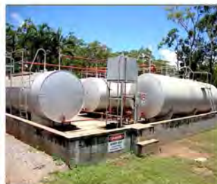
Pirlangimpi Fuel Storage
