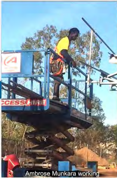
Ambrose Munkara working on edge protection
