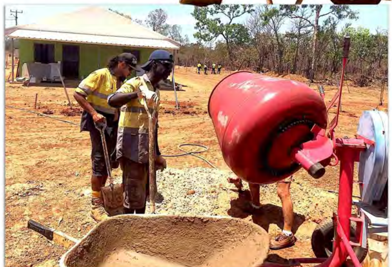
Daniel Portaminni and Ambrose Munkara at construction site
