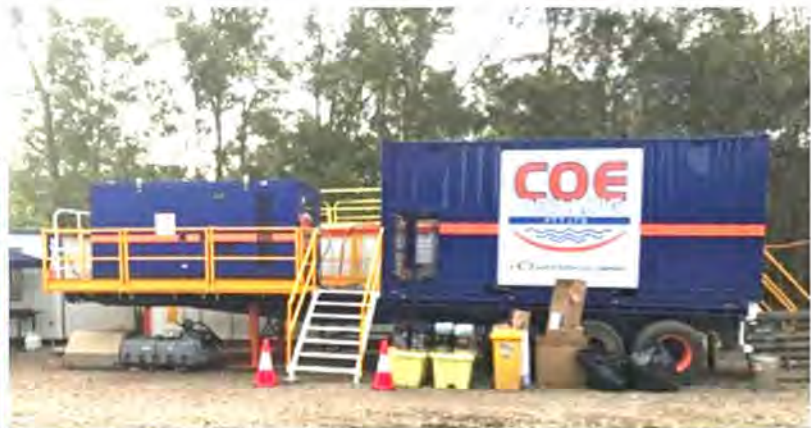
Photo: A similar drill rig will be used.
