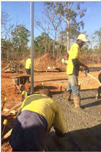
Building verandah slab on Lot 928
