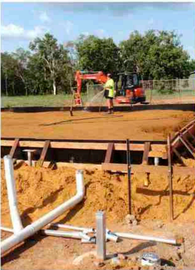
Foundation for the bulk store
