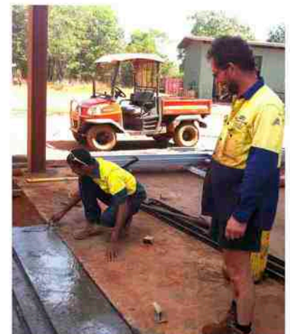
Tiwi and PMP workers laying the ground
