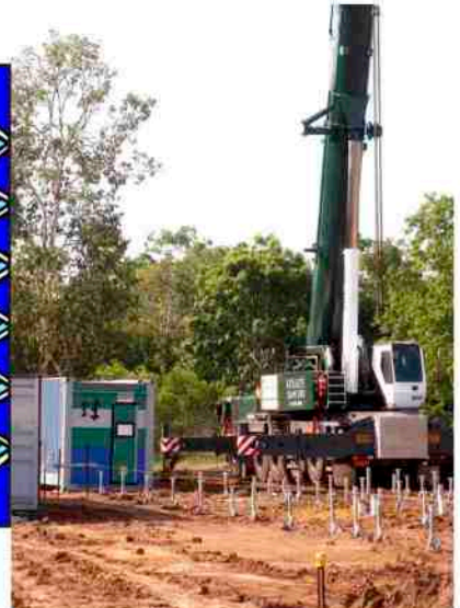
First unit placed by crane
